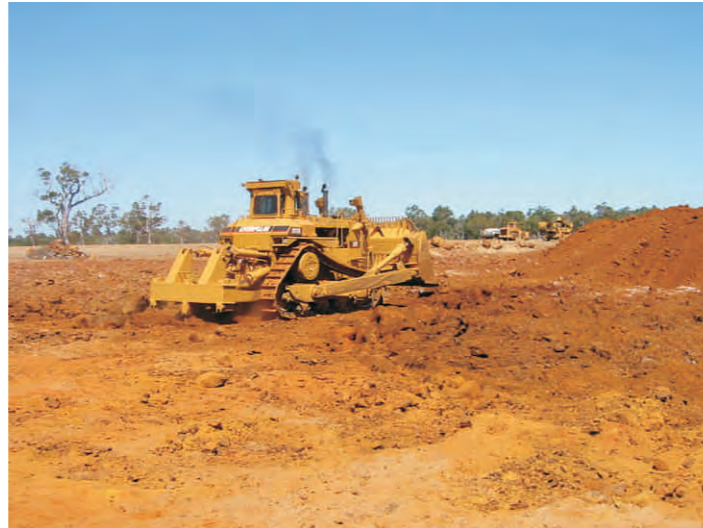
Catalano bulldozer opening new ground
