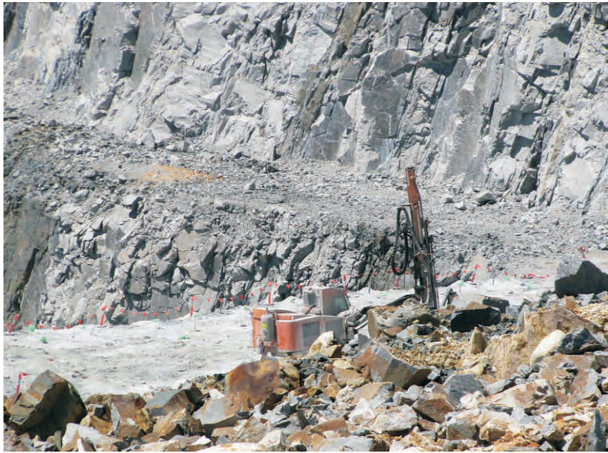
Drilling blast holes
