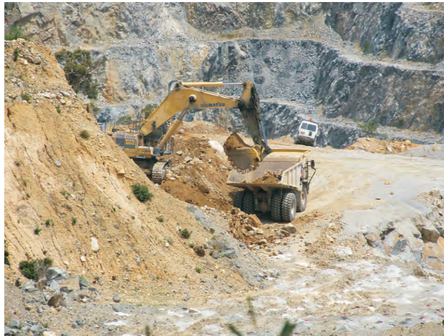
Excavation loading a small haul truck
